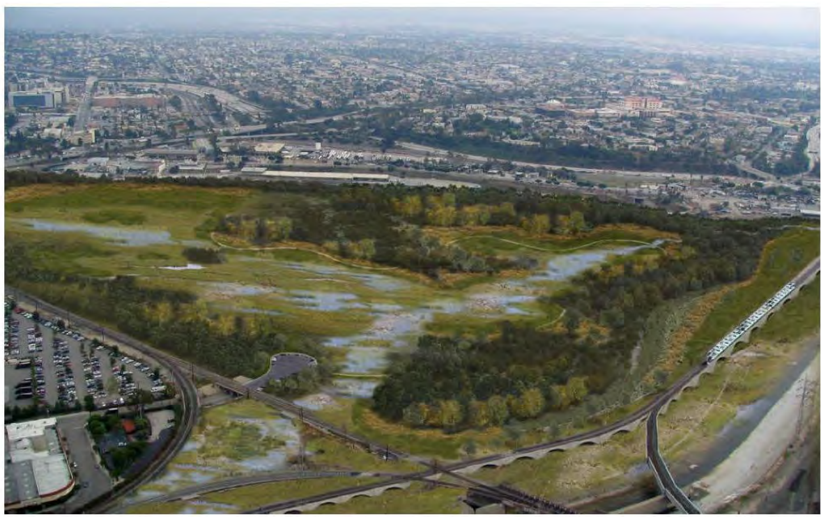
Figure 4-30 Reach 8. LATC, Looking Southeastward (Existing and Rendering of Proposed Restoration Measures) 16
