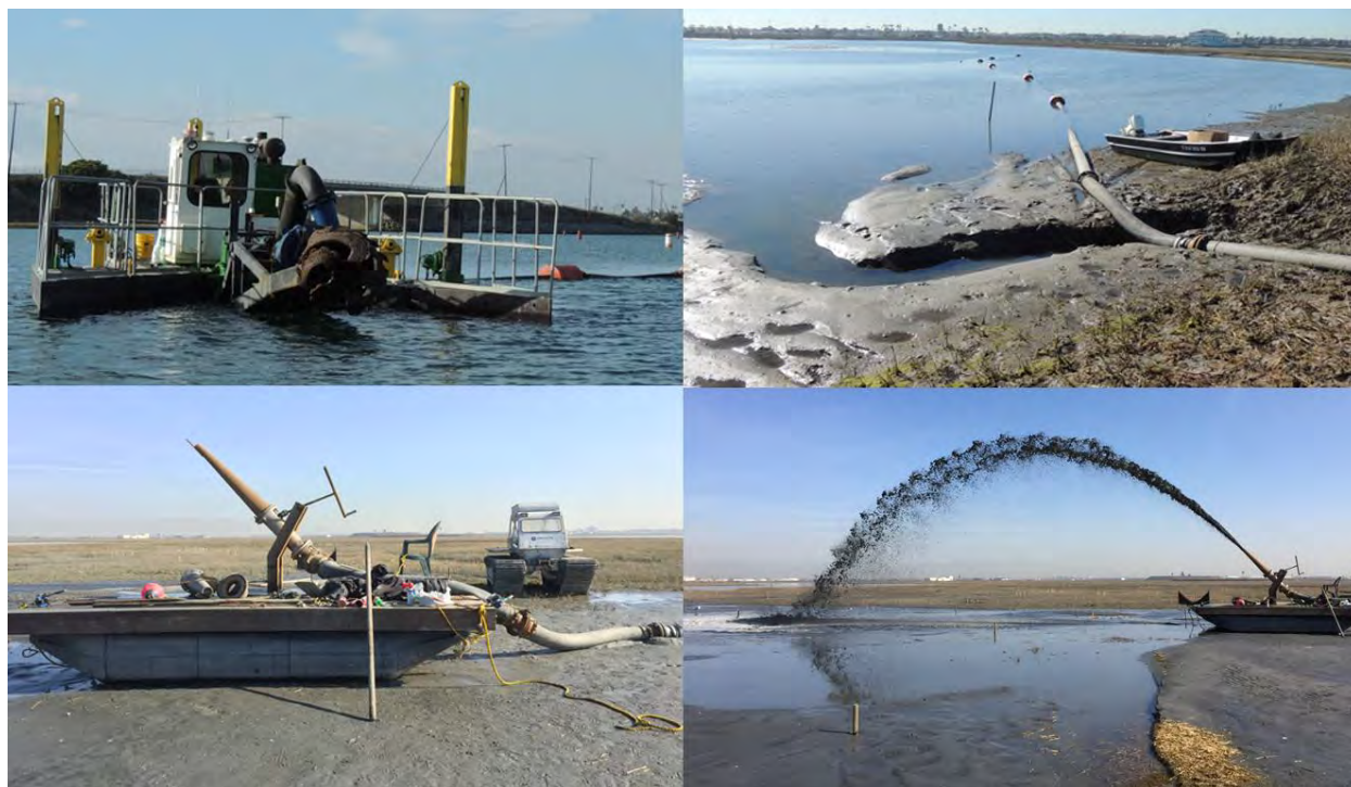
FIGURE 13. THIN LAYER SEDIMENT DEPOSITION CONSTRUCTION METHODS
