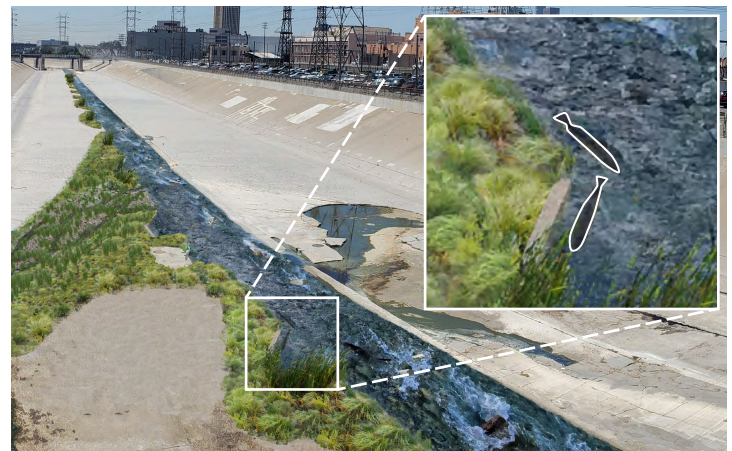
Proposed design for Reach 8A that will help steelhead travel upstream by increasing water depth, slowing flows, and creating deep resting pockets. (Source: Stillwater Sciences)
