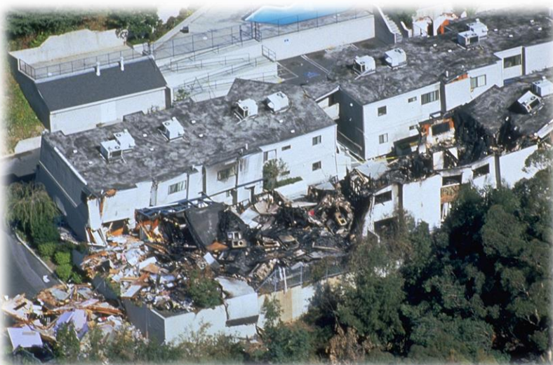
Photo: Soft Story Building Collapse at Northridge, California, Source: FEMA Photo Library
