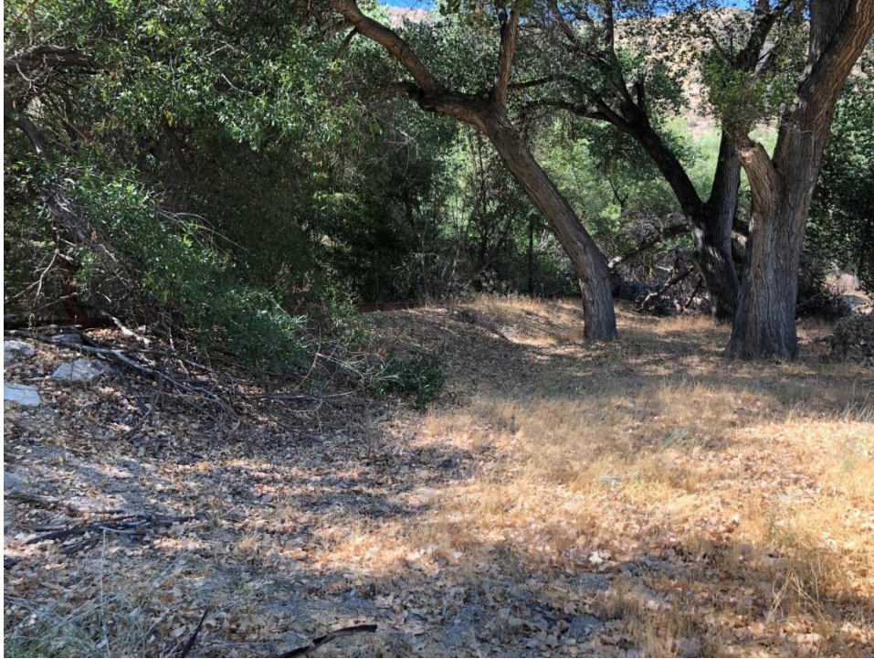
Photo 3. Berm and flood wall to be removed with graded hummock to preserve and support native trees (see 00 00 03 Grading Plan).
