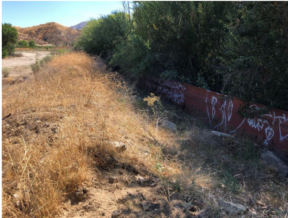
Photo 2. Looking northeast along berm and sheet metal wall to be removed.
