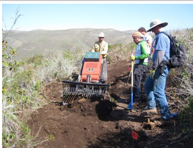
A trail dozer or Bobcat loader would be used to make an initial trail cut due to their small size, maneuverability, and ability to avoid native habitat and biological resources.
