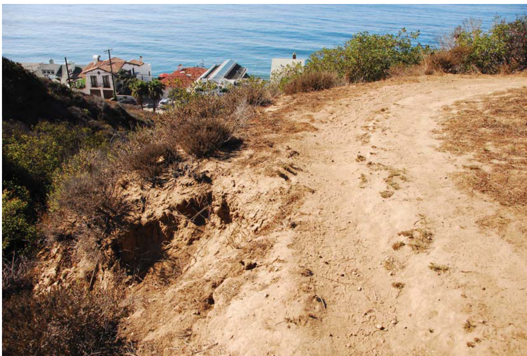
Photo 15 - Erosion encroaching into existing trail along blufftop.
