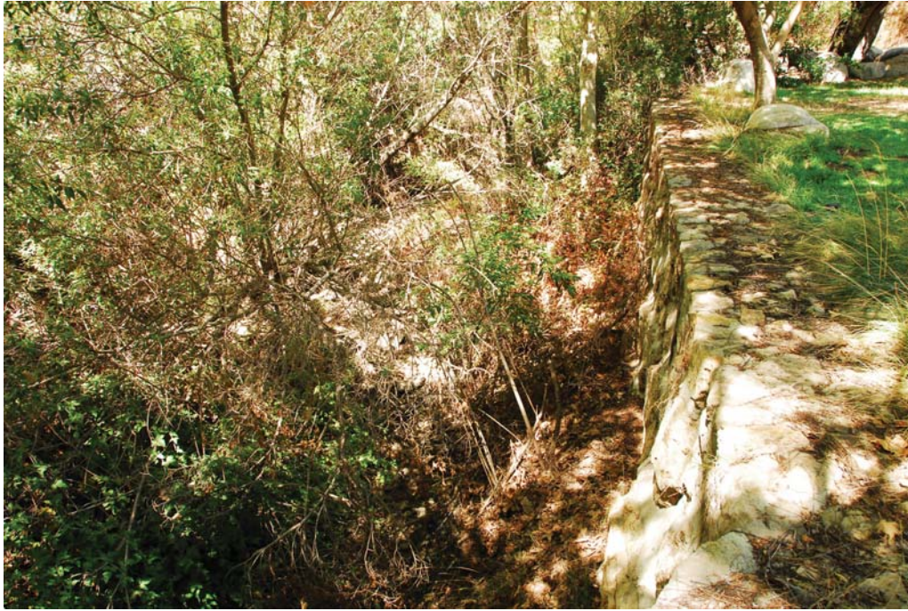
Photo 9- View looking north along rock retaining wall on east bank of Ramirez Canyon Creek at proposed bridge crossing. Wall is about 7 feet high, and is located about five feet above the streambed.
