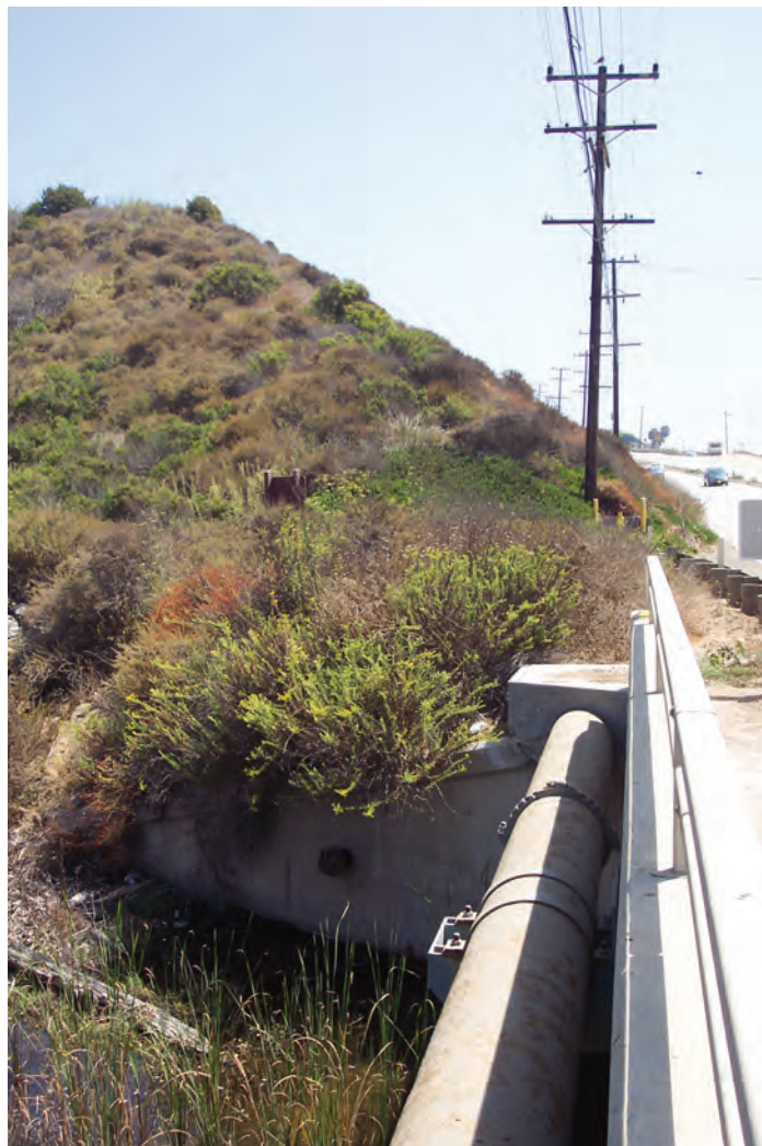
Photo 1 - Water line, retaining wall and road fill at proposed trailhead parking area at Pacific Coast Highway at Corral Canyon.
