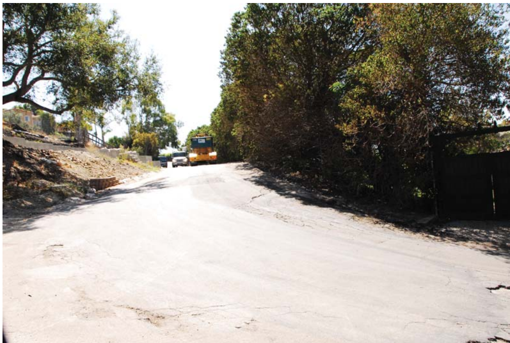
Photo 13- View looking south along upper section of Delaplane Road. Slopes ascend and descend from the edge of the existing pavement at a gradient of about 2:1.
