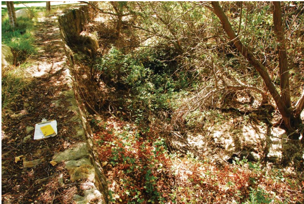
Photo 10 - View looking south along rock retaining wall on east bank of Ramirez Canyon Creek at proposed bridge crossing. Creek encroaches within about five feet of the wall.
