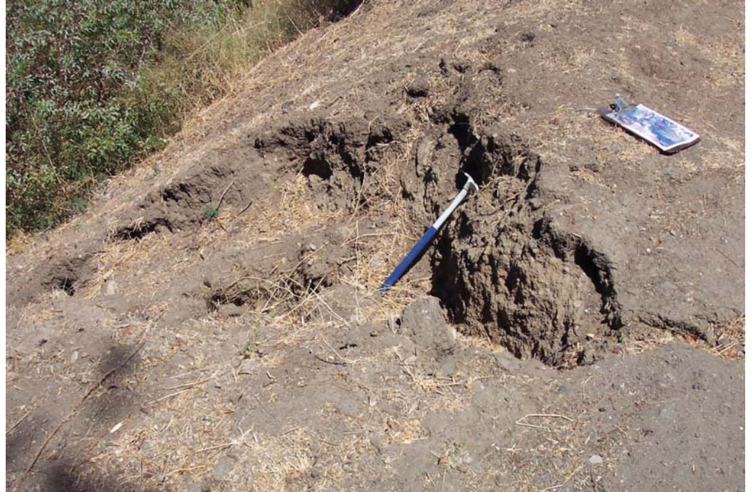
Photo 6 - Erosion due to concentrated drainage across existing maintenance road at Escondido Canyon between trailhead and ADA Camp Area.
