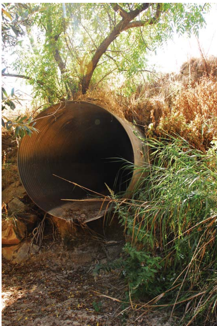
Photo 7 - Outfall of pipe that carries flow along Escondido Creek below crossing for access road. Surrounding fill is eroded to a steep angle to vertical.
