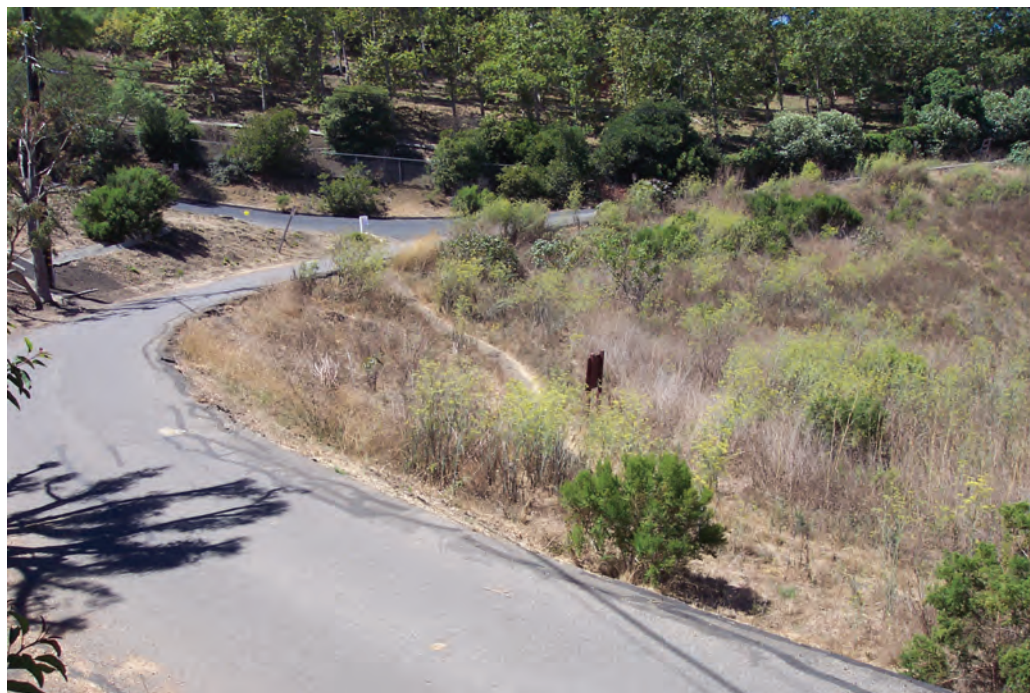
Photo 4 - Vicinity of proposed 15,000 sf parking area near trailhead at Escondido Canyon. Constructing parking area may require substantial grading. Road cracks suggests fill settlement and possible downhill creep. The road and descending slope were resurfaced prior to September, 2009.
