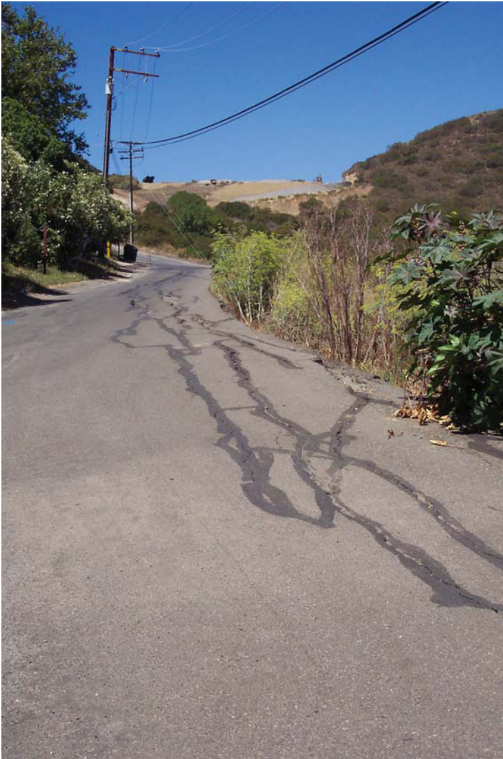
Photo 5 - Closer view of cracking along Winding Way. The outer five to ten feet of the roadway are affected. Road was resurfaced prior to our site reconnaissance in September 2009.
