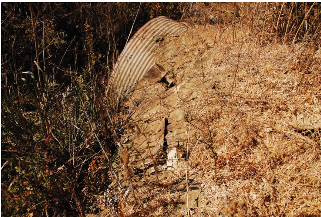
Photo 8 - Inlet to pipe that carries flow along Escondido Creek below crossing for access road. Note fill contains debris including old tracks from heavy equipment.
