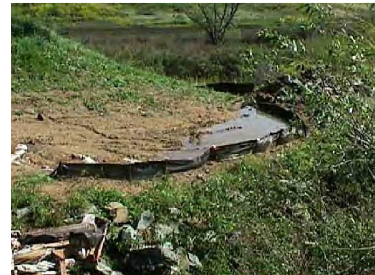
INSTALLED SILT FENCE
