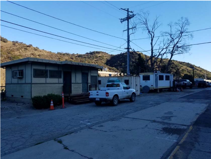
View of the existing structures and utilities on the Project site
