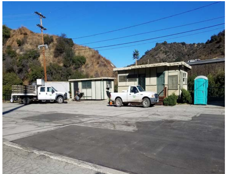
View of the existing buildings/structures, utilities, and currently paved areas onsite
