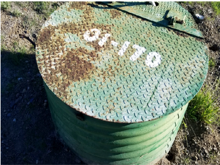
Photograph of an existing monitoring well onsite
