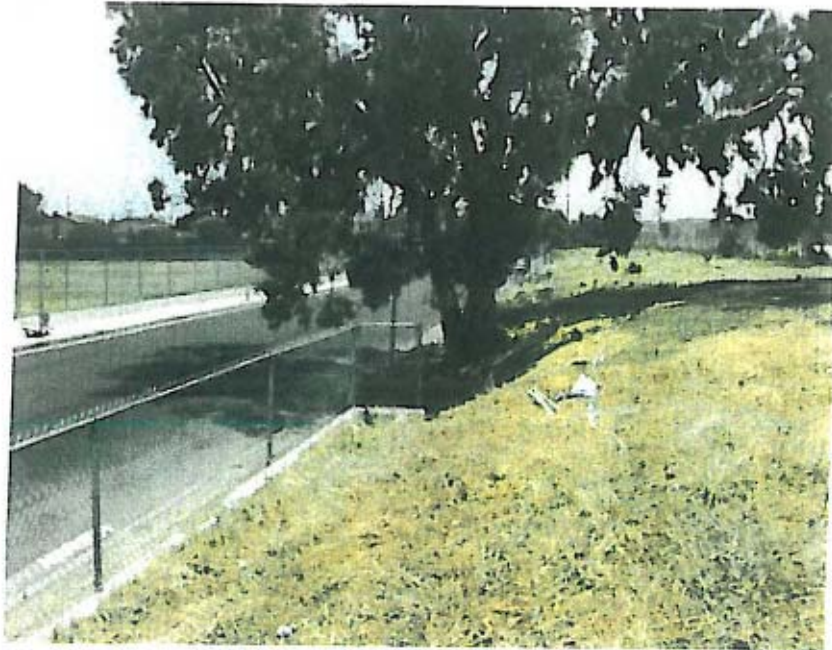
Photograph 1 – Landward Side of Levee Slope
