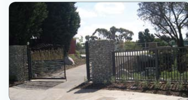
McConnell Avenue Gateway
