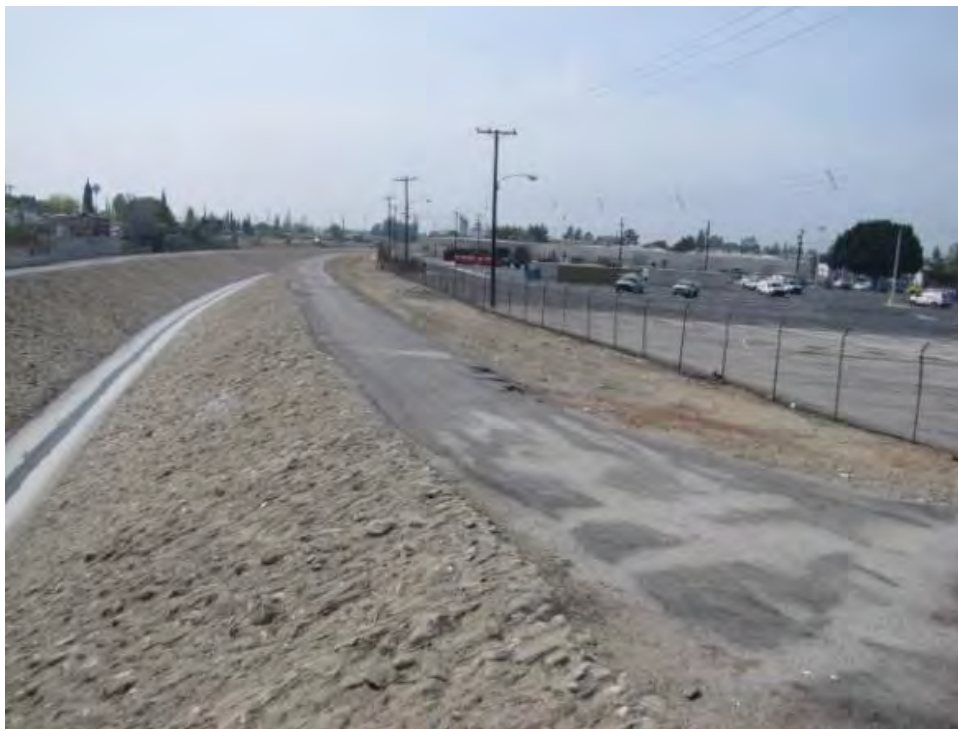
View of Pacoima Wash from 5th Street looking southwest
