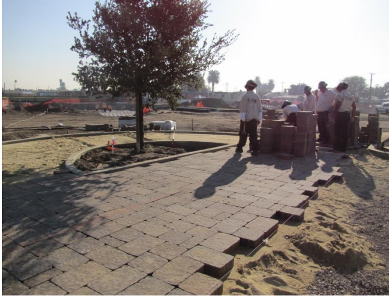
Current progress as of 11/2/11
