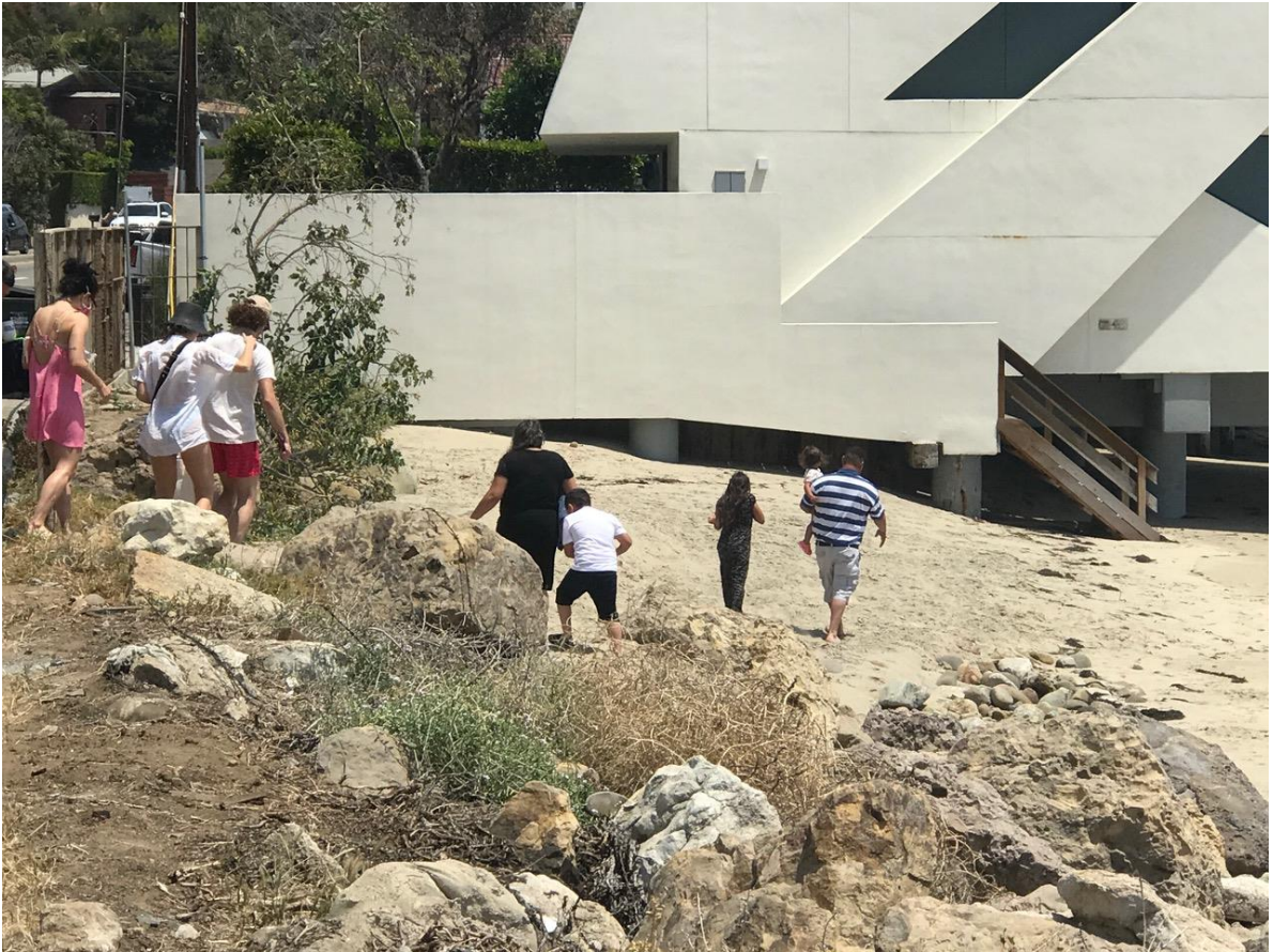
Photo 6: View of existing fence at 21704 PCH on May 8, 2021
